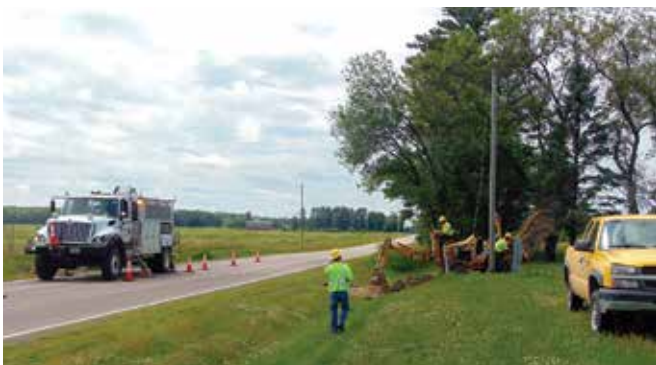
Pictured here and at the top is the safety instructor from Dairyland Power Cooperative conducting a safety inspection of one of our crews in the field.
